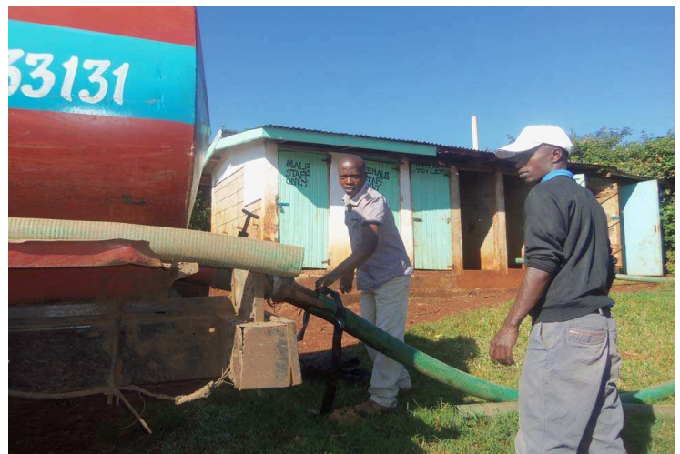
Sanitation and Hygiene (Exhauster emptying the school toilets)
